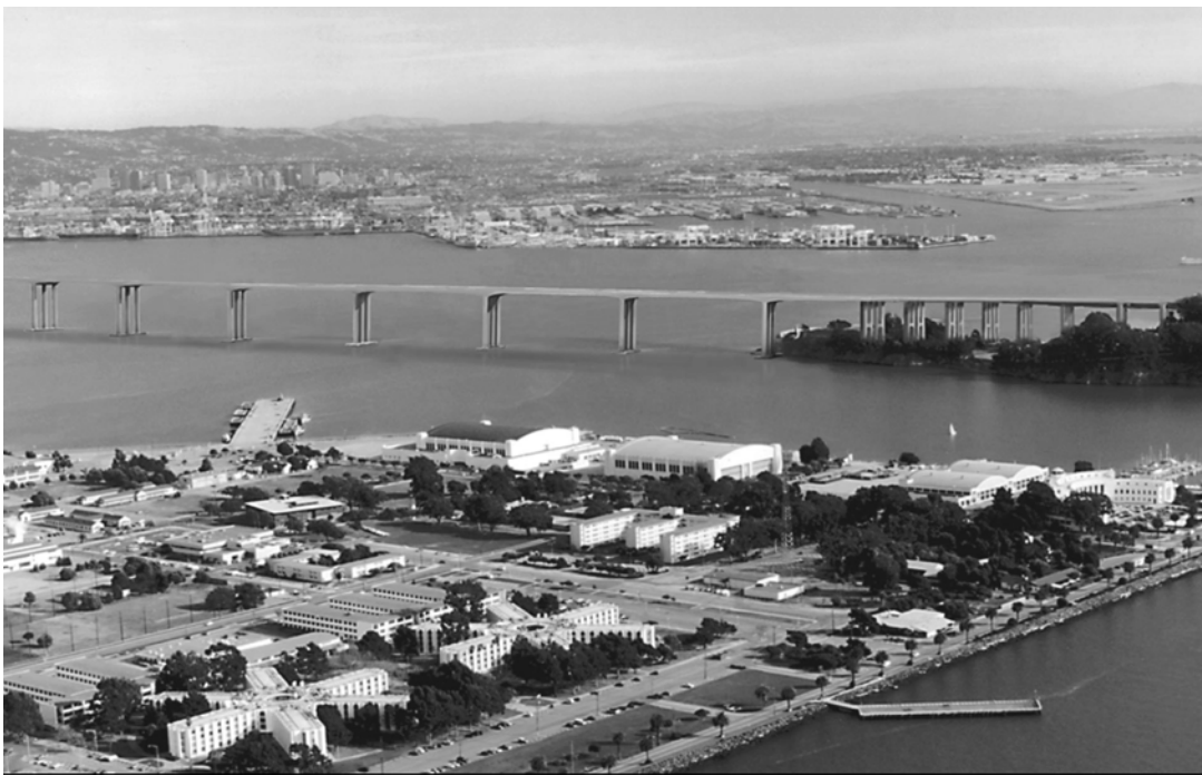
Artist's rendering of the basic viaduct-style east span proposed by Governor Wilson (sometimes referred to as the “skyway” design). Subsequent designs will incorporate a suspension section with tower over the navigation channel adjacent to Yerba Buena Island.
